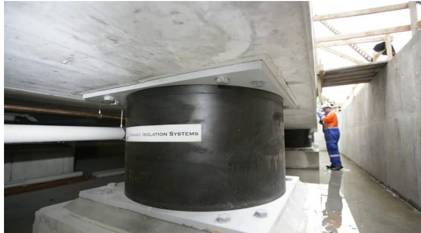
Figure 4: Base Isolation for a Building
